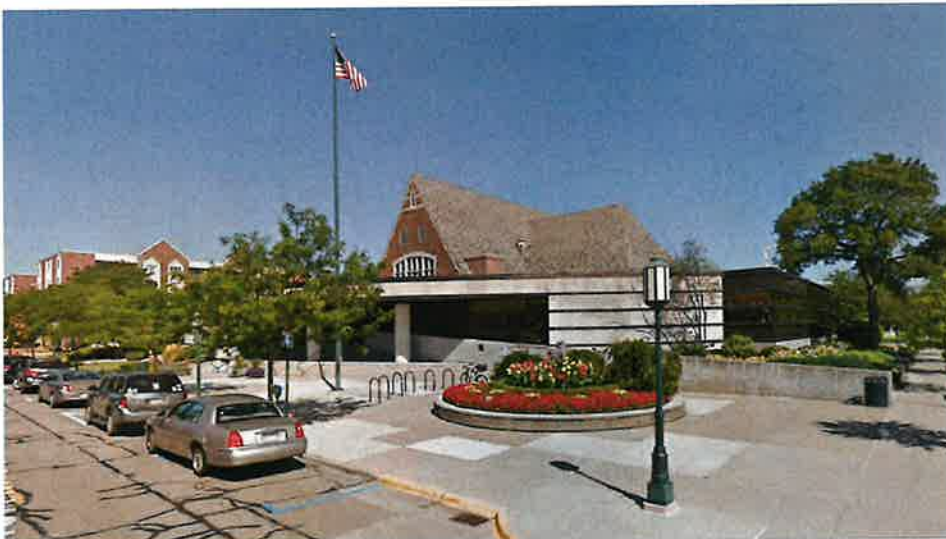
Figure 46. The Library's entrance plaza.
