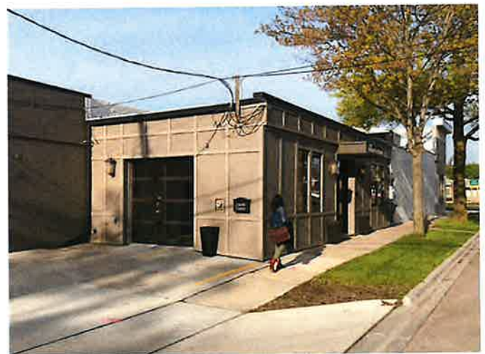
Figure 54. Building with potential for sleeve activation.
